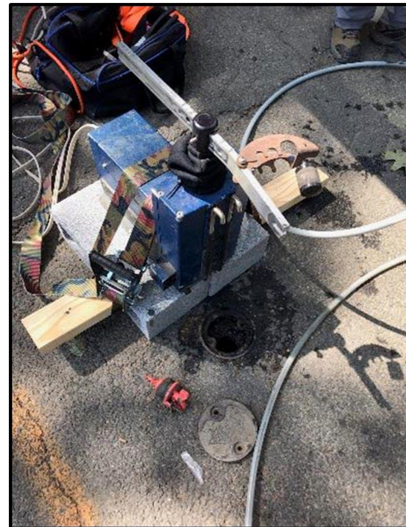
Groundwater sampling well
